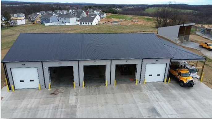
Public Works Building
